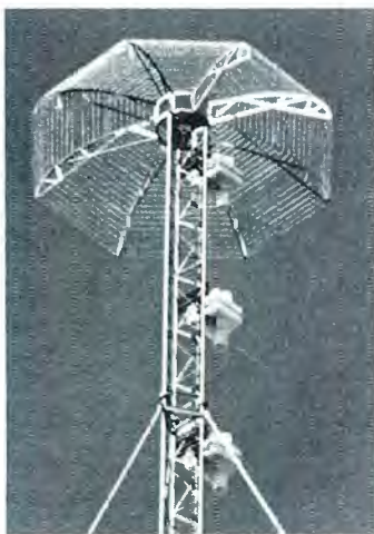
LEA LIGHTNING BARRIER. Typical Hemispherical Dissipation Array in use at a broadcast site.
